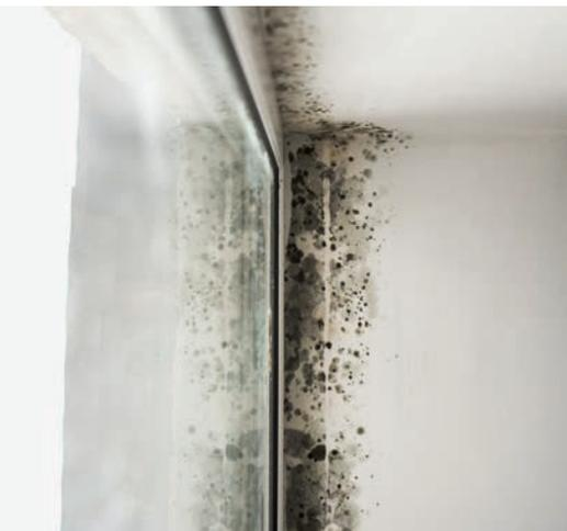
PHOTOGRAPHED EXAMPLES OF TYPICAL MOULD CAUSED BY CONDENSATION
